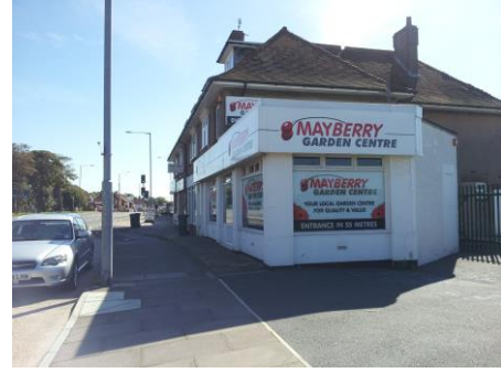
Existing retail units north east of site.
