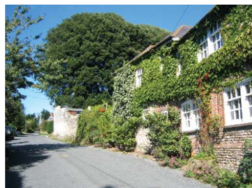
Flint houses in Patching
