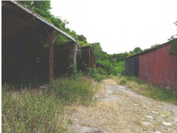
1. View from southern entrance showing disused open sheds along the western side and one of the barns in the centre. Grid ref. TQ14820569. Direction north.
