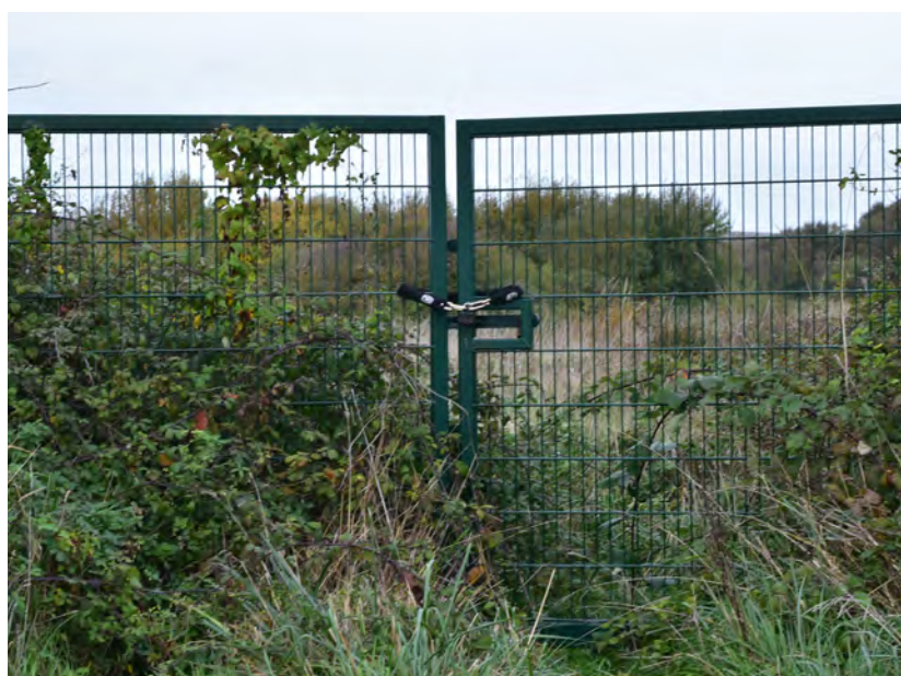
The site is enclosed by security fencing, including a locked gate
