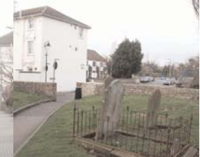
Poor frontage onto St Mary's Churchyard
