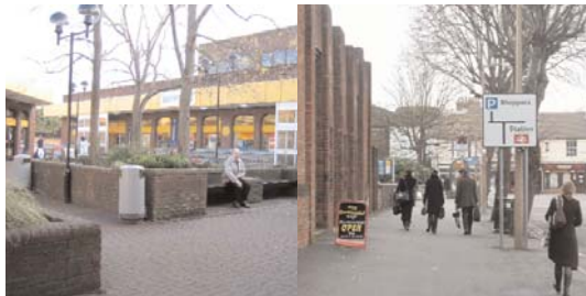
Small retail precinct around the entrance to Somerfield turns its back to Ham Road Ham Road suffers from an inactive edge
