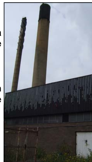
Fig. 25: Boiler house and chimneys
