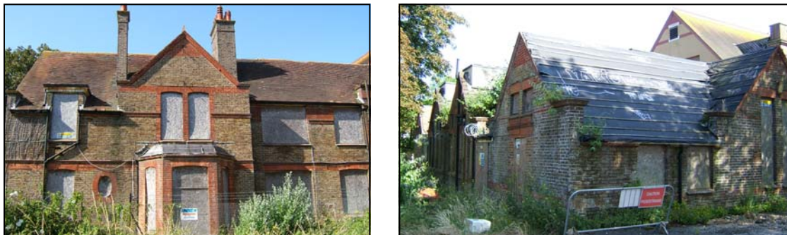
Figs. 12 & 13: Secondary halls (south elevation) and kitchen block
